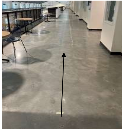
Figure 1. Testing Site: Level 2 of ERB in Statesboro, GA.
