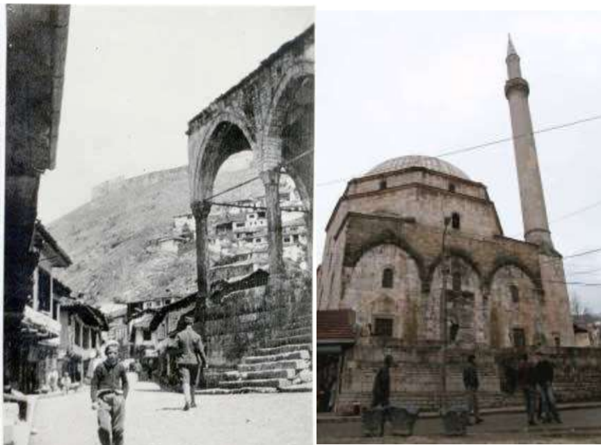
Figure 6. The porch before demolition, 1918.
