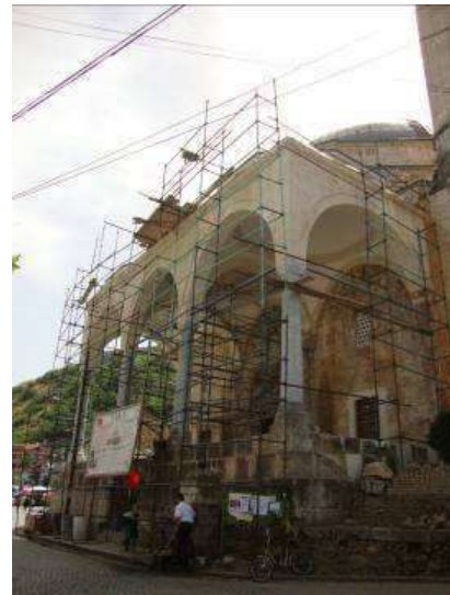
Figure 17. Completion of the construction of
